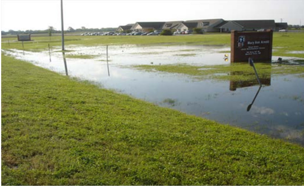
Figure 6.16. Standing water south of Sections 8 through 13B in May 2011.
