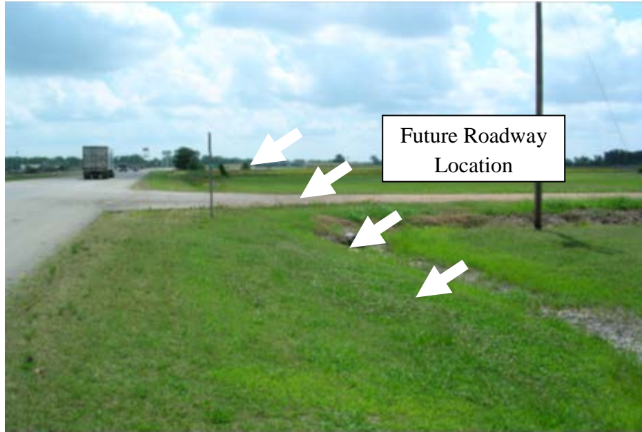
Figure 3.5. Test site prior to construction (Howard 2006).
