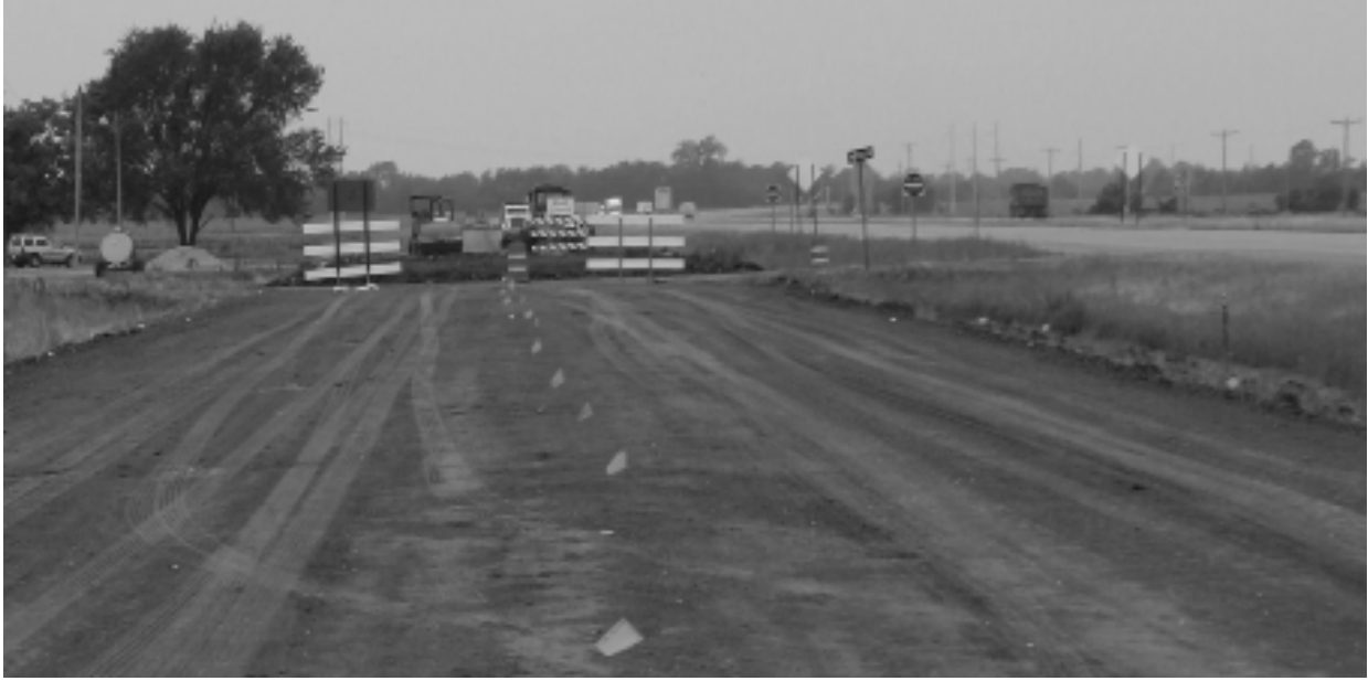
Figure 3.10. Finished cut subgrade (Howard 2006).
