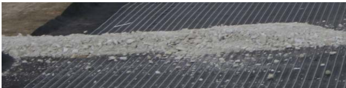
Figure 3.16. Crushed stone covering fine sand, geosynthetic strain gage, and cable (Howard 2006).
