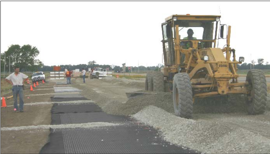
Figure 3.18. Lateral placement of crushed limestone on geosynthetics (Howard 2006).
