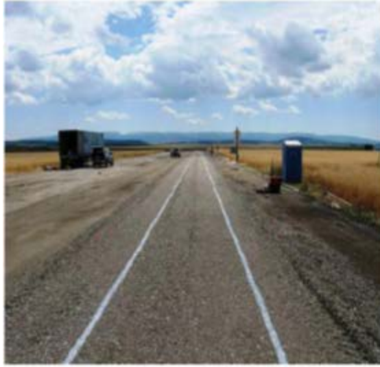
Figure 2.6. Full-scale field testing (Cuelho and Perkins 2009).
