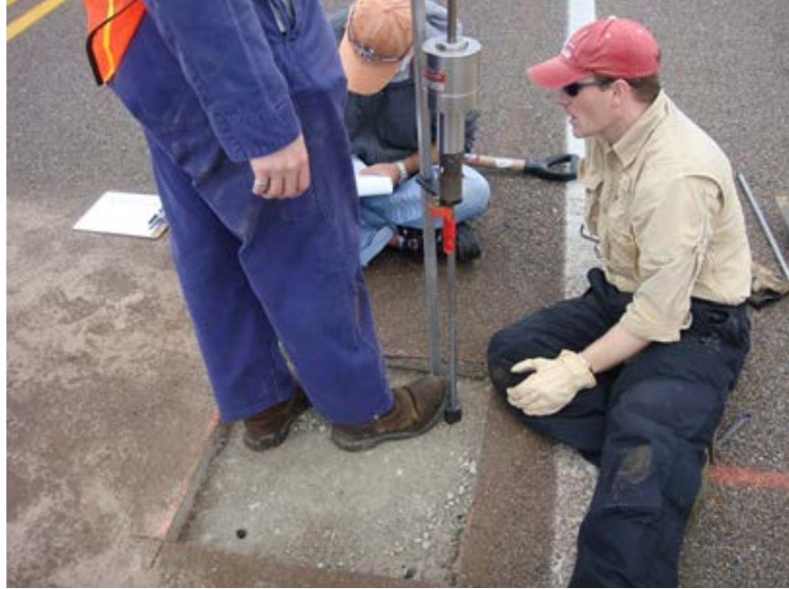
Figure 6.5. DCP test conducted in southeast corner of excavation area of Section 13W.
