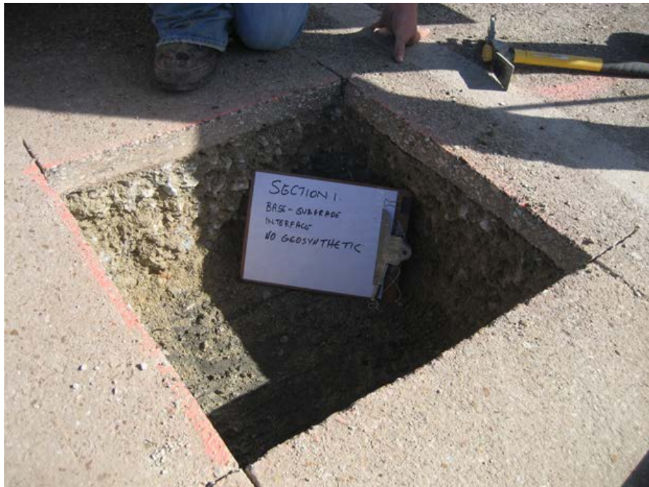
Figure 6.8. Base-subgrade interface of Section 1 (no geosynthetics).
