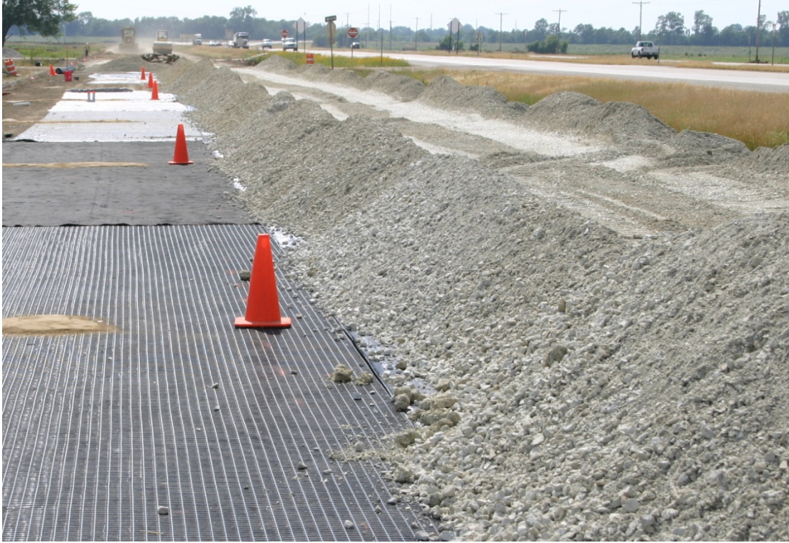
Figure 3.17. Base course placement on non-instrumented lane (Howard 2006).
