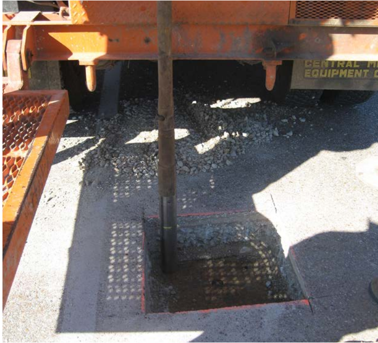
Figure 6.10. Shelby tube pushed in southwest corner of excavation area.
